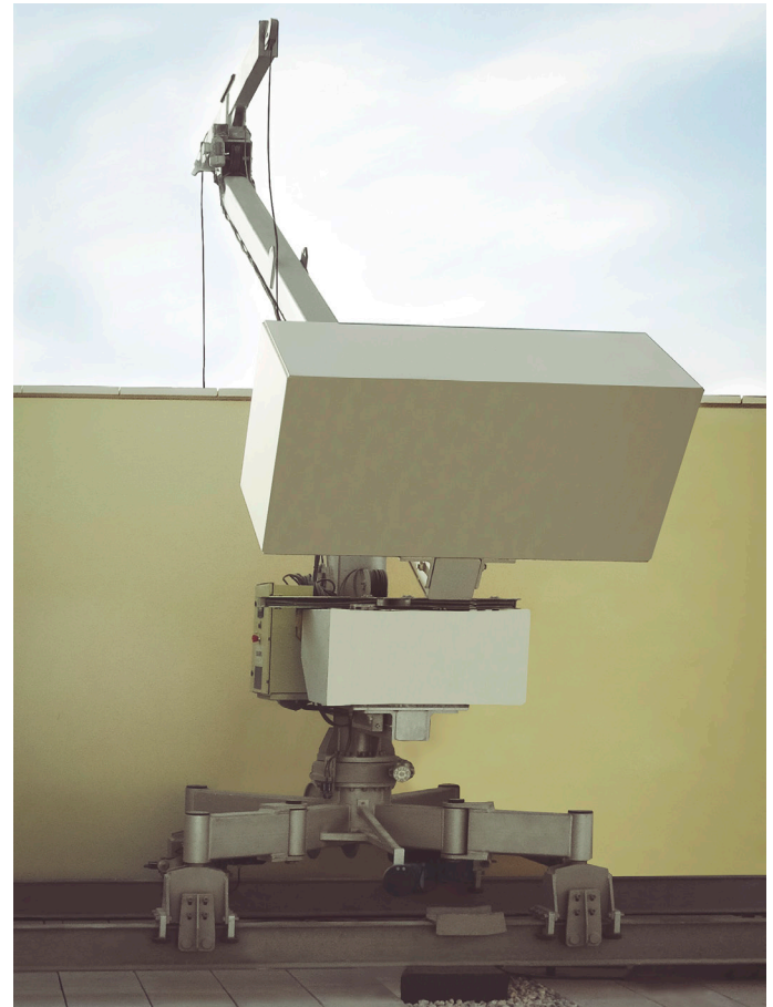
FBA 1 with jib luffing, in order to pass the cradle over the high parapet. Installed in Doha, Qatar.
