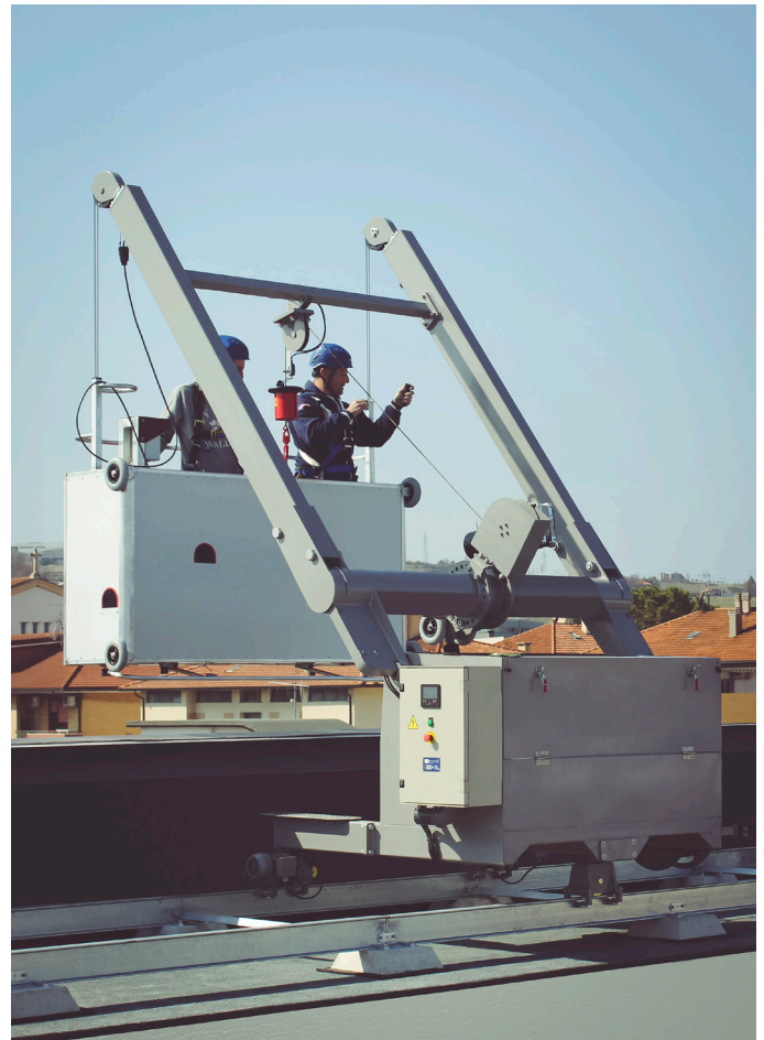
BMU FBA Type 2: the standard lightest machine.
