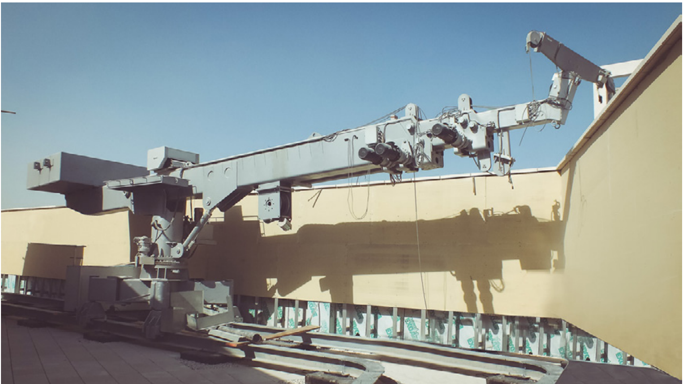
FBA Type S - P16: BMU with Telescopic jib, slewing arm, luffing device and auxiliary hoist.
