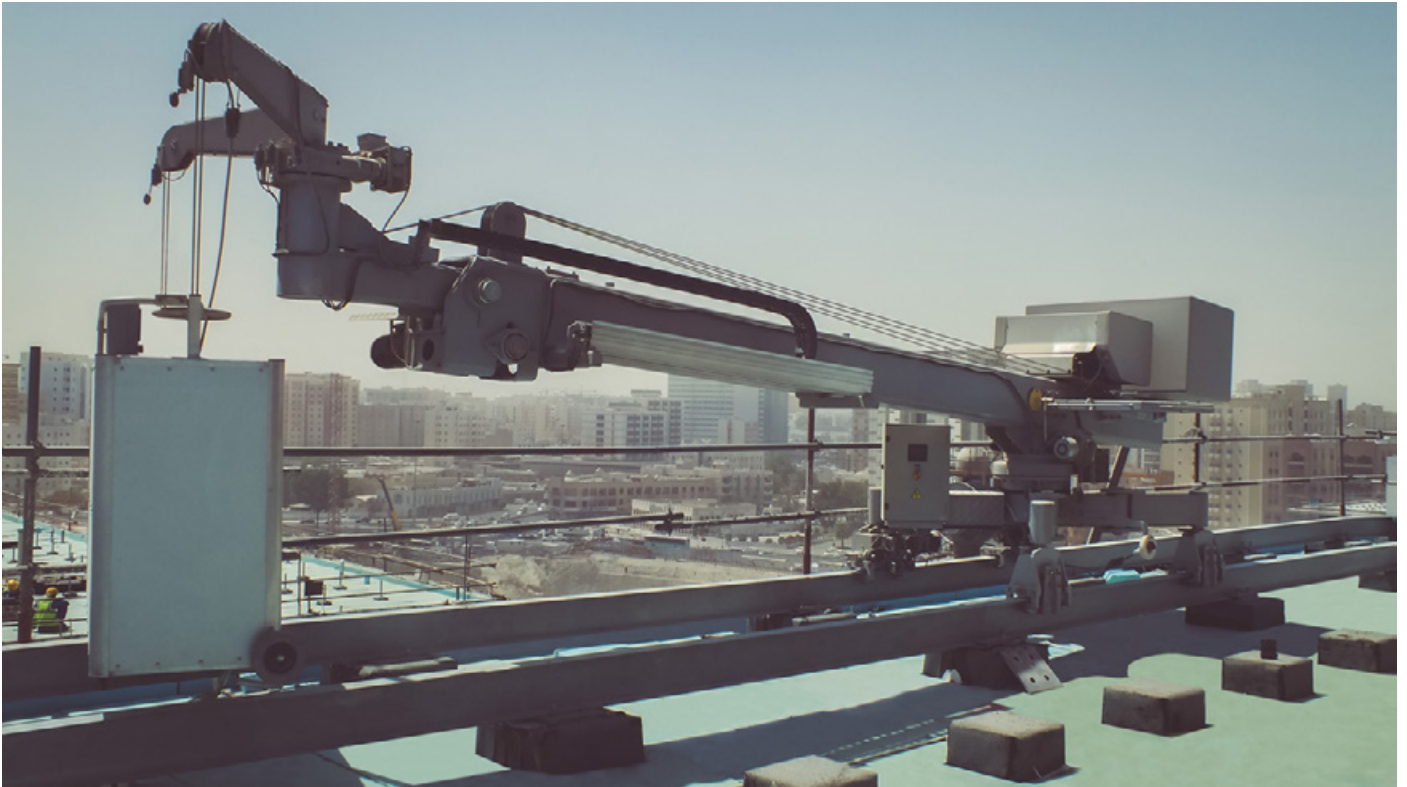
FBA Type S - S03: BMU with telescopic jib, slewing arm and auxiliary hoist.
