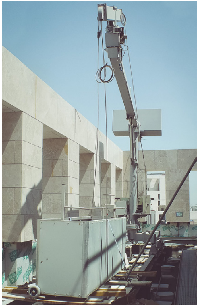
FBA Gomyl BMU Type 1 - U06 with one jib.
