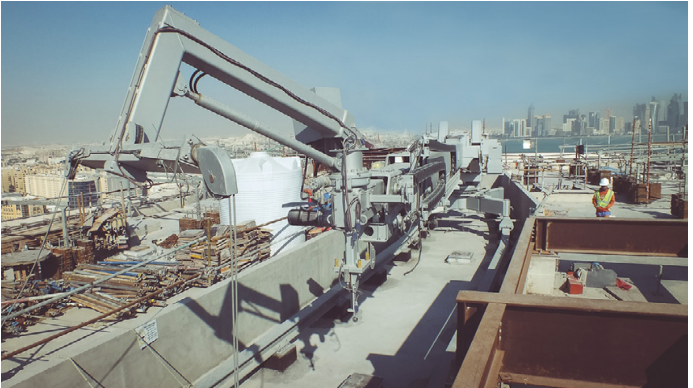
FBA Type S - T08: BMU with Telescopic jib, slewing arm, luffing device, luffing spreader bar, telescopic mast -scissor type- and auxiliary hoist
