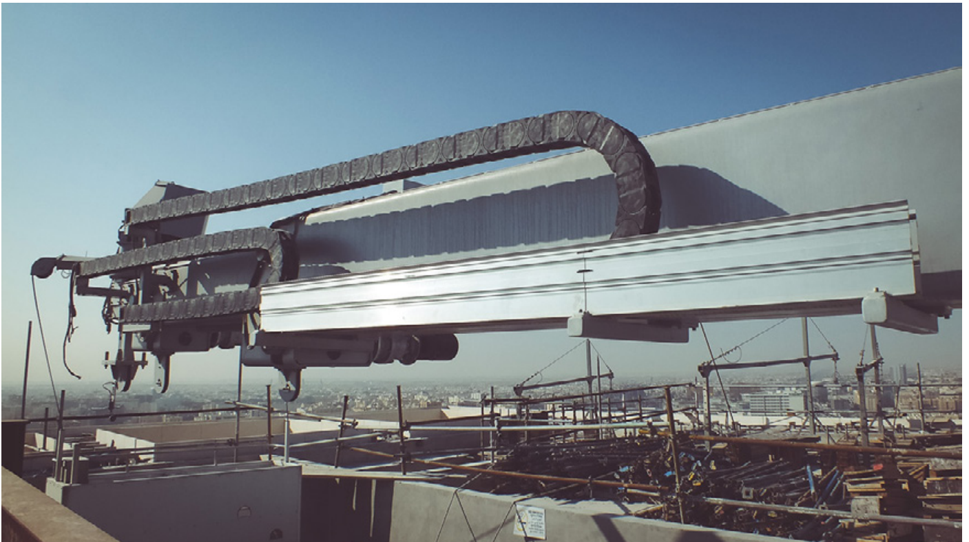
FBA Type S - T08: BMU with Telescopic jib with spreader bar in parking position.
