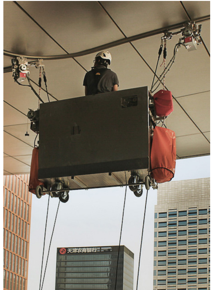
Cradle RopeClimber suspended by 2 battery powered trolleys.
